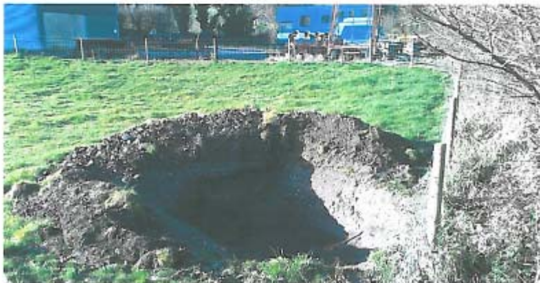
Hole dug in field (by others) opposite Farncomb Farm – note water in base
